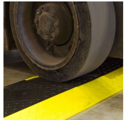
Pic. 6.3.2 Cables under yellow jack
