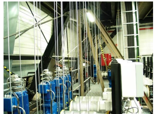
Pic. 10.3.11 Fly bar motors
