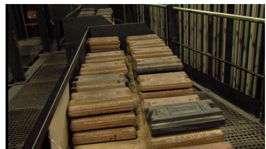
Pic. 3.3.11 Counter weight table
